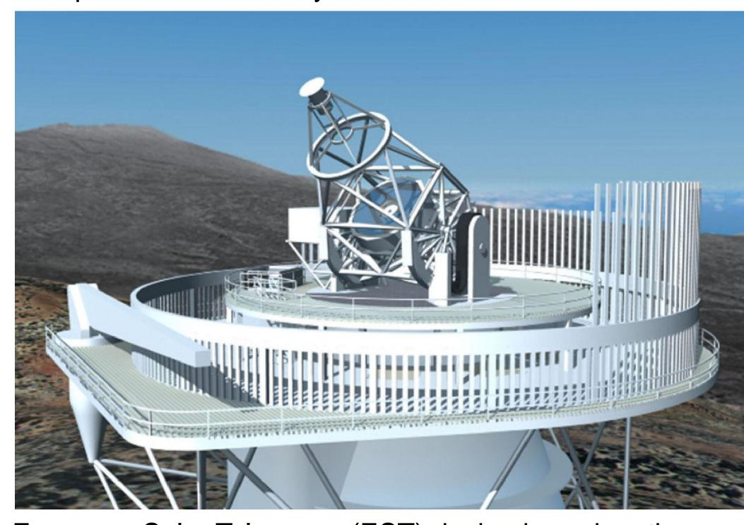
European Solar Telescope (EST) design based on the open principle with open telescope structure and completely open-foldable dome specialised for observations with highest resolution of polarised light for understanding the Solar activity.
