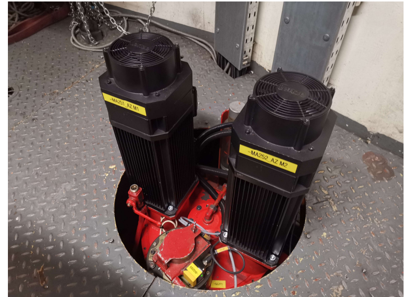
Left Azimuth Motors
