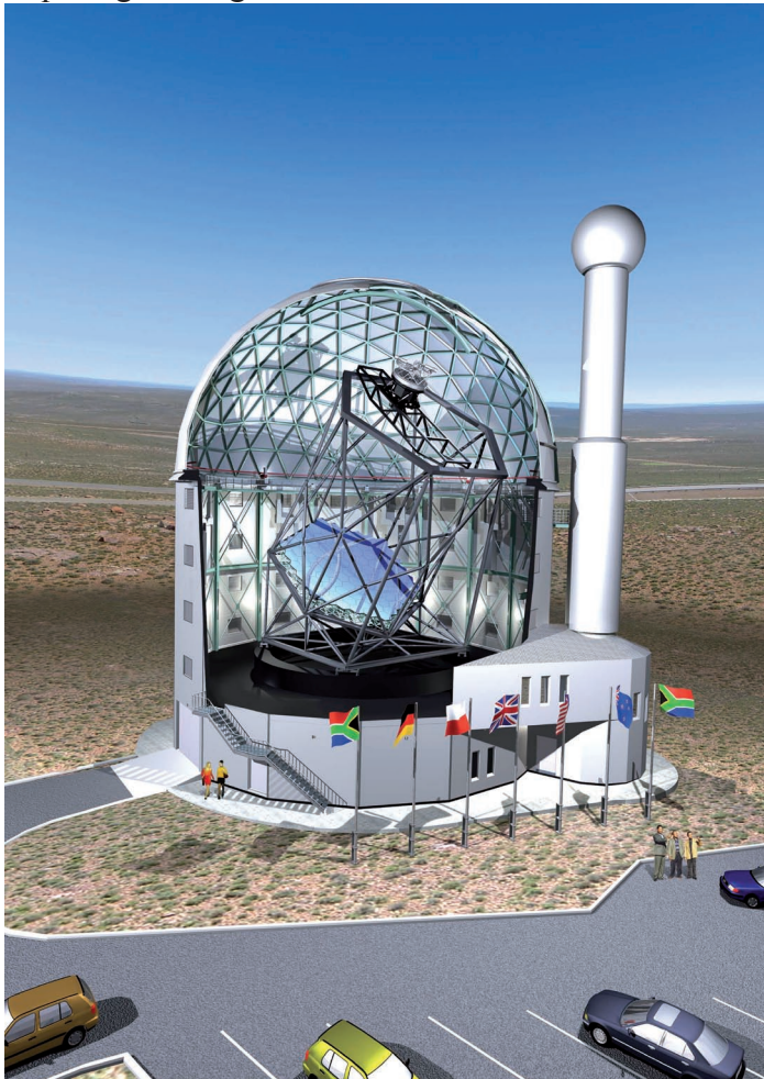
Figure 2: Cutaway schematic of SALT and its environs, showing the key elements of the segmented primary mirror, which can rotate in azimuth, but is at a fixed elevation of 53^\circ , and the Tracker (which carries the instrument payload). Image courtesy SALT Foundation.
